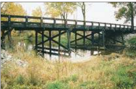
Pipe Creek Bridge
