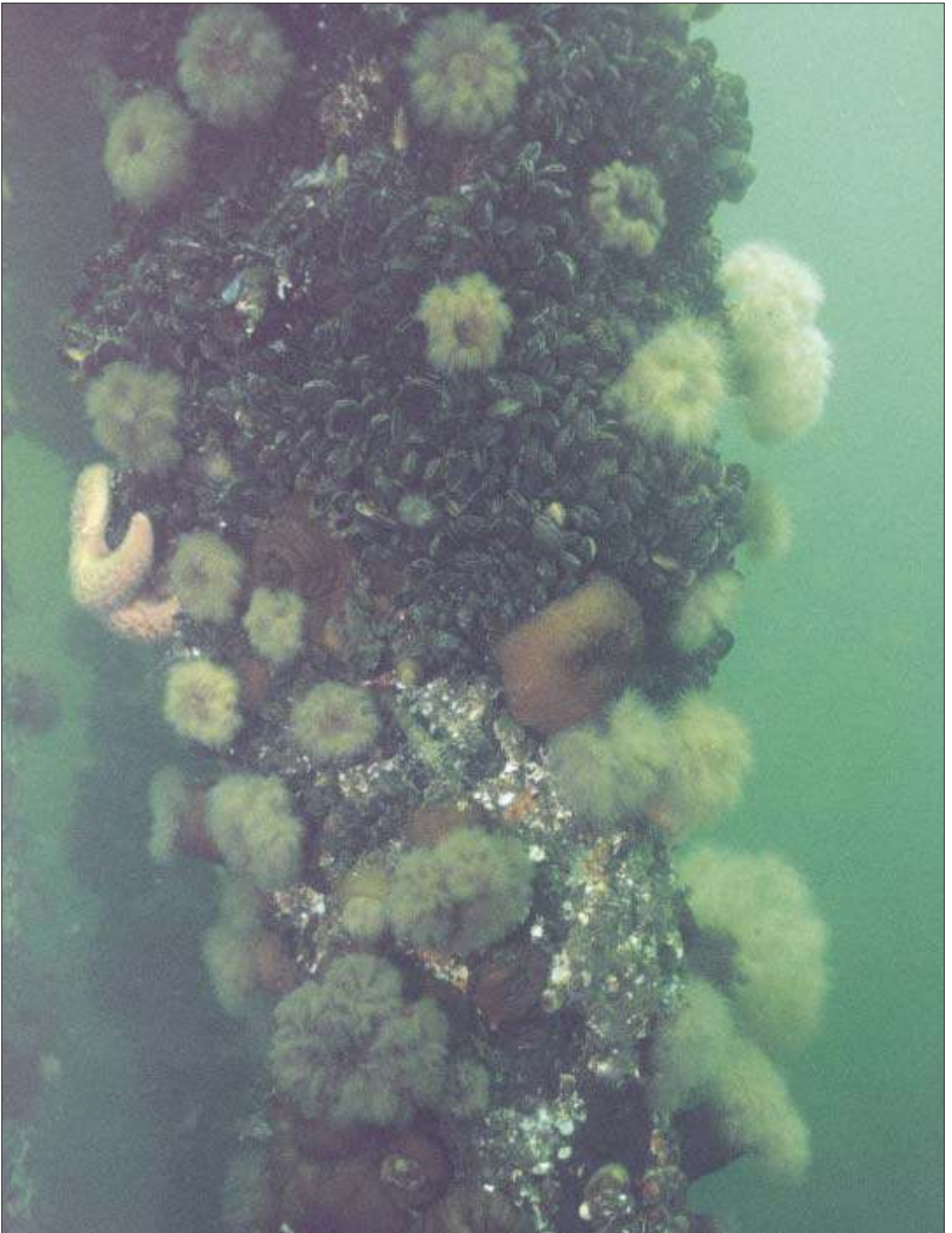
Invertebrate community growing on a new creosote-treated marine piling in Sooke Basin
