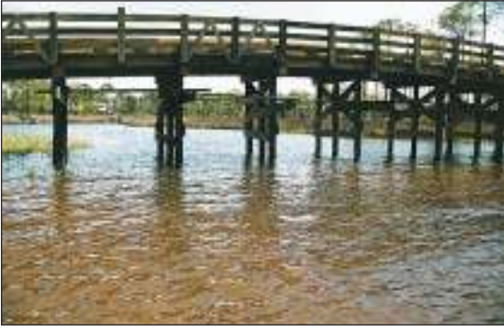
Horseshoe Bayou Bridge
